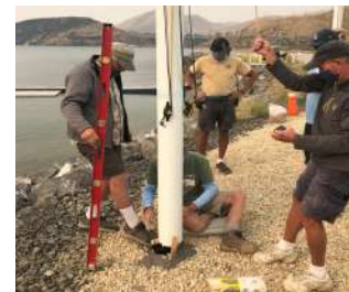
Shade sail masts under construction.
